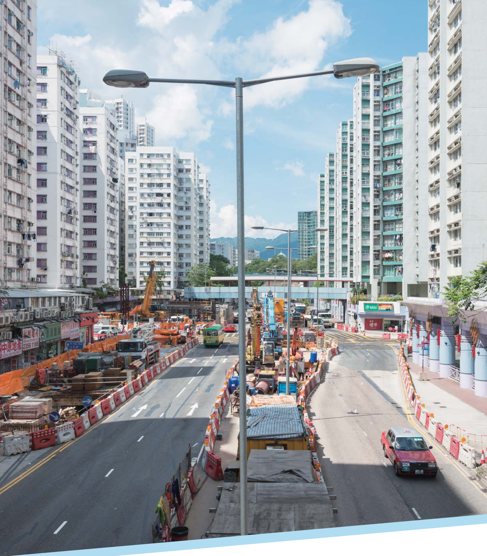
MTR Contract No.1002 - Kwun Tong Line Extension: Whampoa Station and Overrun Tunnel 港鐵合約編號1002 — 觀塘綫延線：黃埔站及避車隧道建造工程
