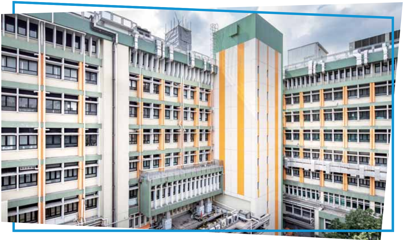
Main Contract for Refurbishment of Hong Kong Buddhist Hospital 香港佛教醫院翻新工程總合約
