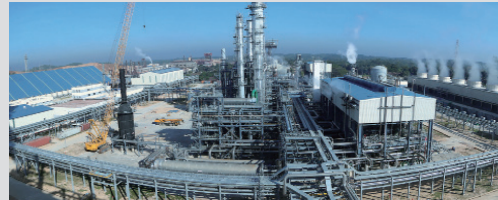
孟加拉沙迦拉化肥厂获得中国建设工程鲁班奖（境外工程） Shahjalal Chemical Fertilizer Plant in Bangladesh won the China Construction Engineering Luban Prize (Overseas Project).
