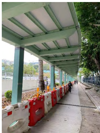
Construction of Walkway Cover
