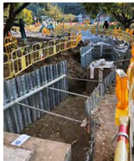
Construction of Sewage System
