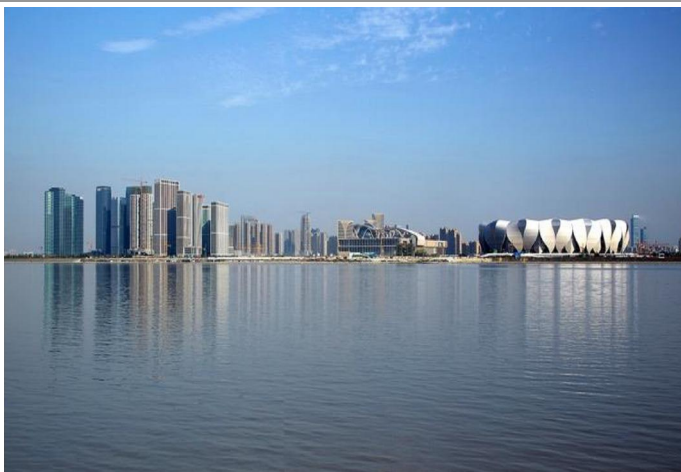
Exhibit 13: Actual picture of Qianjiang Century City A
