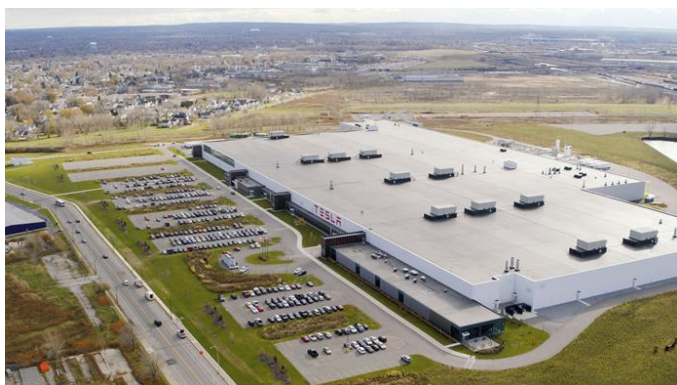
图23: 纽约州布法罗的二号超级工厂 (Gigafactory 2)
