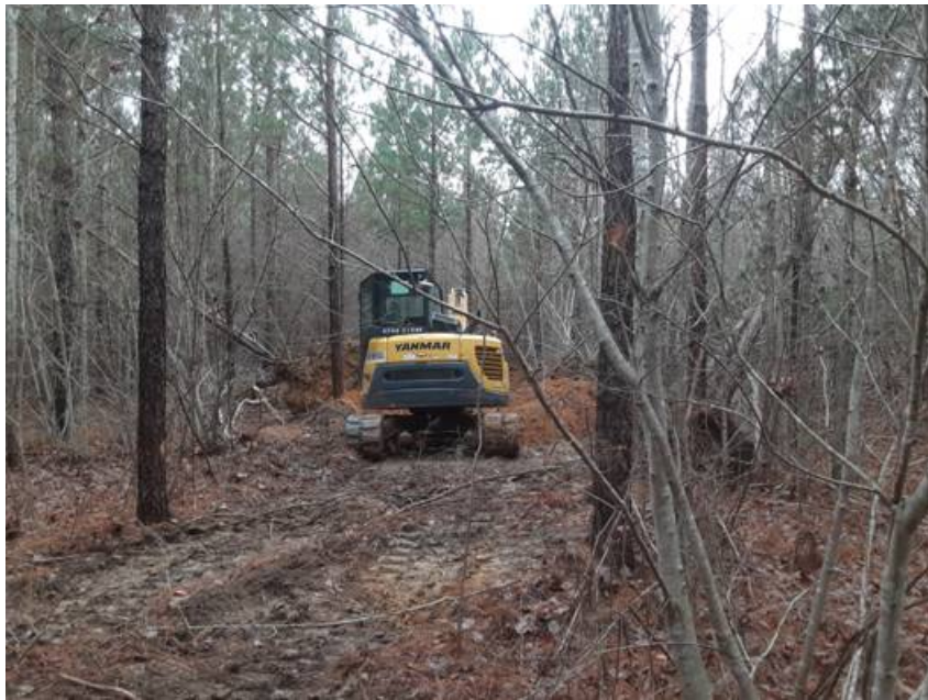
Figure 2: Excavator digging a trench at Argo
