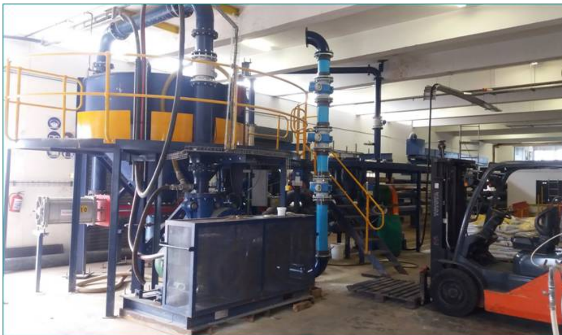
Figure 2: Paterson & Cooke pipe loop facility
