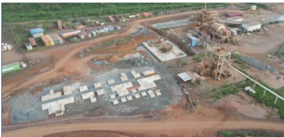
Figure 1: Ball mill and flotation area foundations
