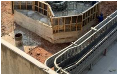
Figure 3: Preparation work at gasifier foundation ahead of final concrete pour.
