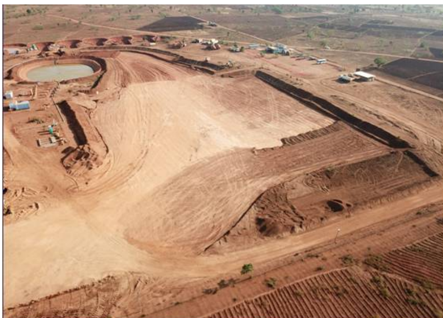
Figures 3 & 4: Test pit during hydro-mining trials (above) and aerial view of test pit being backfilled
