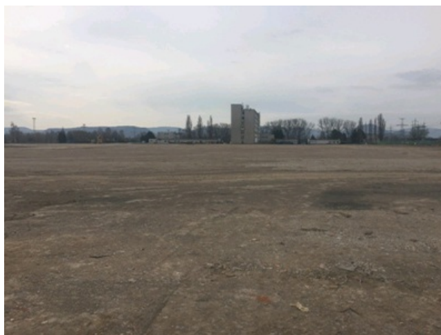
Figure 1: EPR1 site in March 2024 after demolition, clearance and ground rehabilitation. The administration building on the west of the site has been retained and is suitable for use as construction offices.
