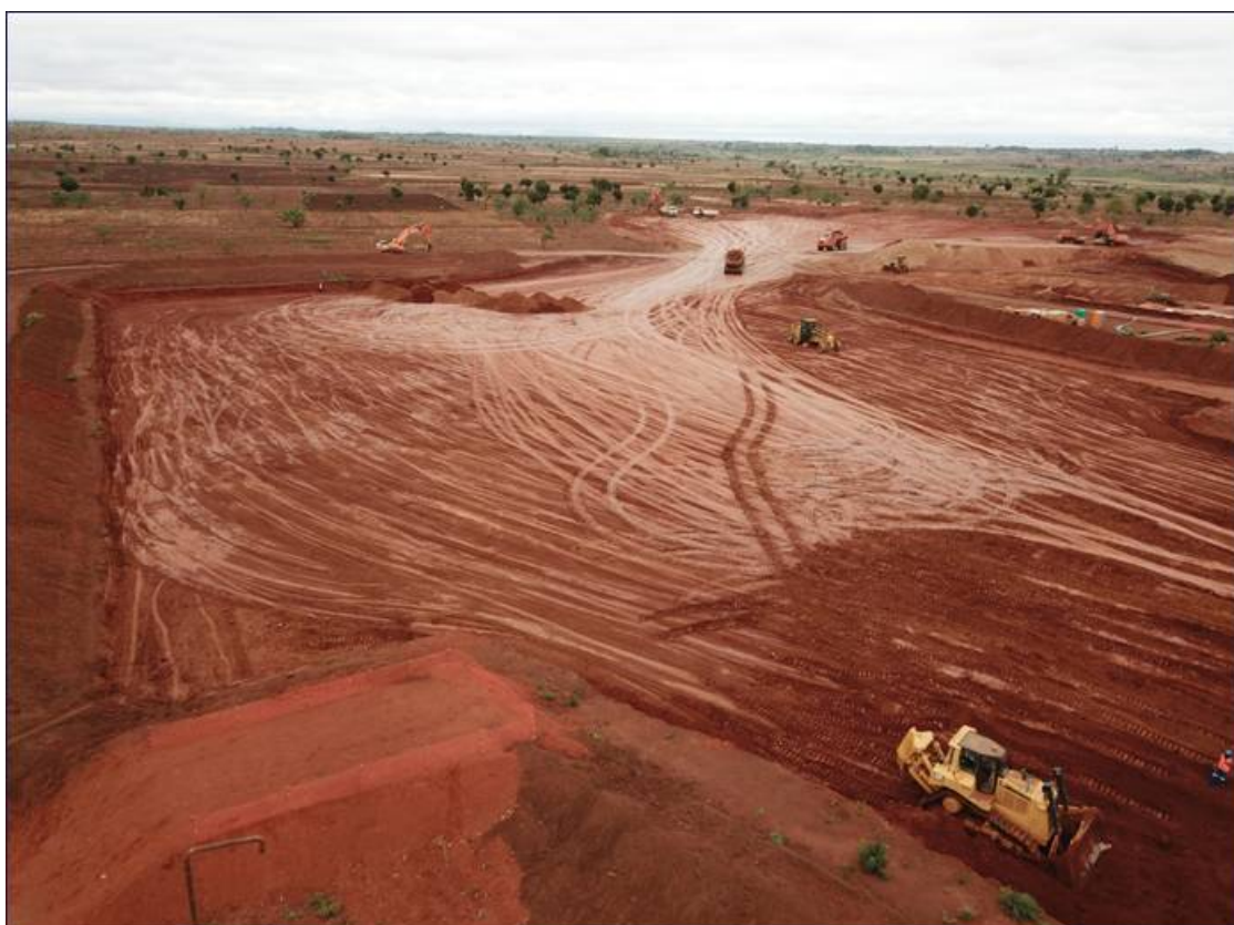
Figure 1: Test pit backfilling
