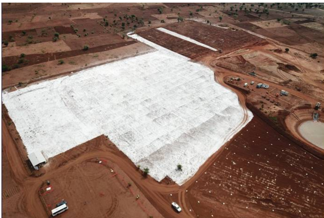
Figure 6: Introduction of lime at the backfilled test pit
