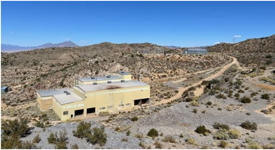
Figure 2: View over the Project's Millsite claims showing the location of the mill (centre), maintenance shack (left), and office/bathhouse, 3000KW substation and water tank (right).
