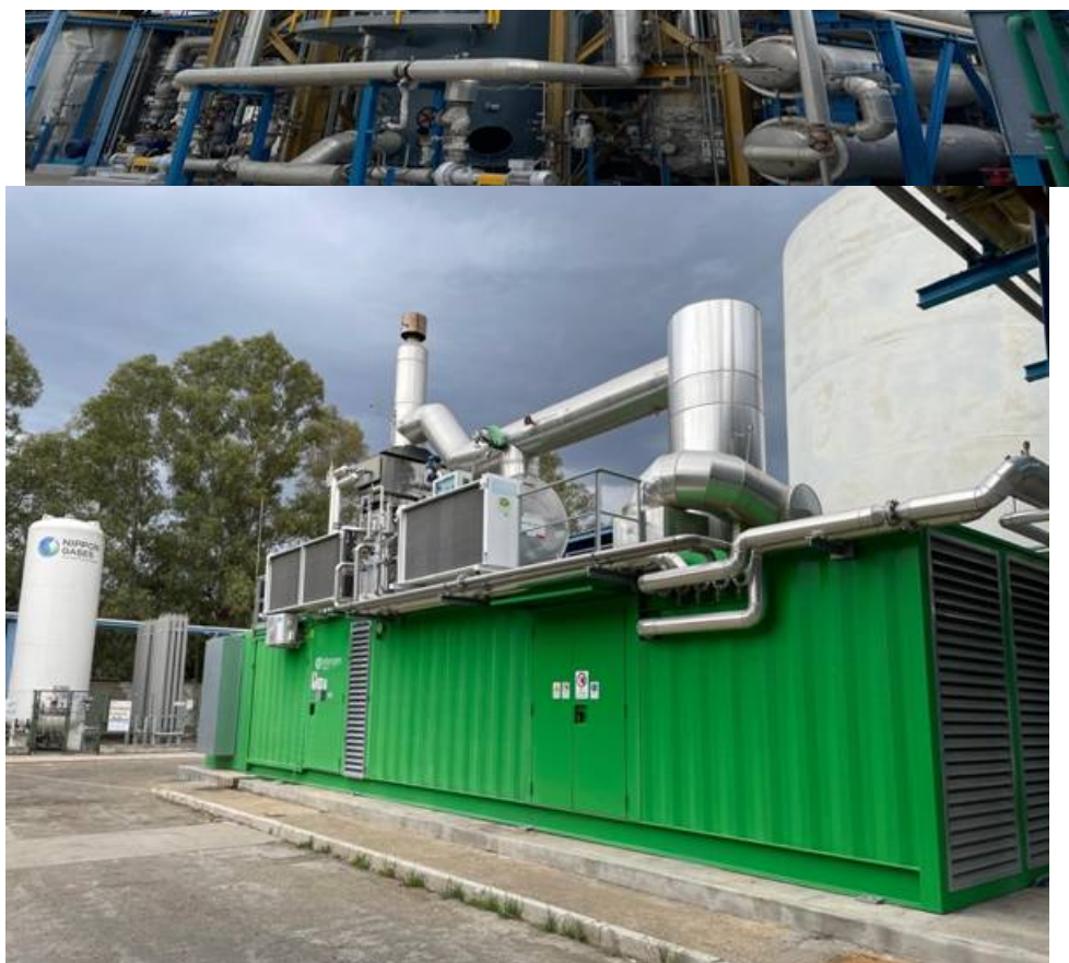
Figure 4 Onsite cogeneration and backup power capacity.
