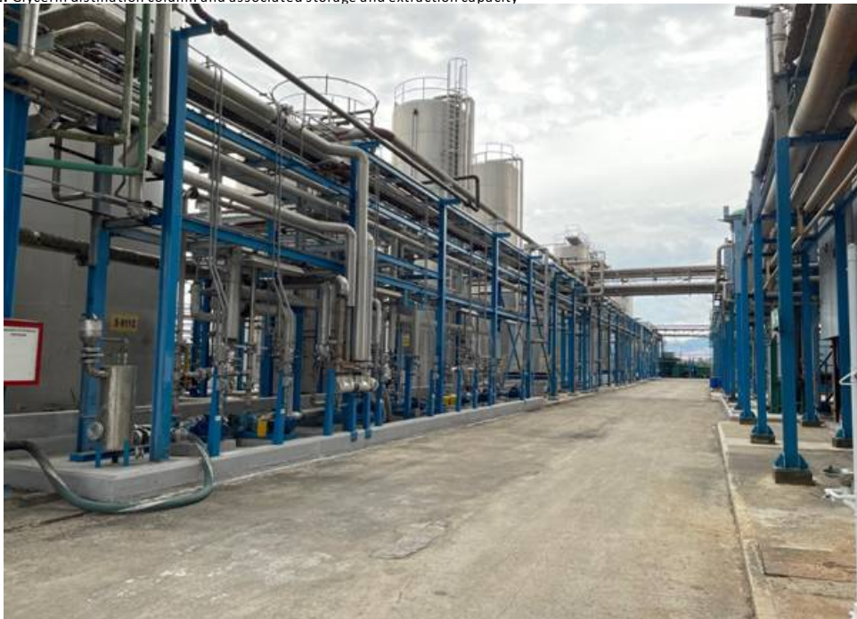
Figure 2. Epoxidized soybean oil storage and extraction facility
