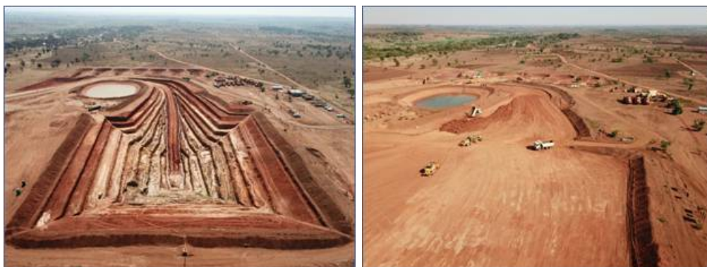
Figure 1: Pilot Phase test pit during mining trials (left) and subsequently backfilled (right)
