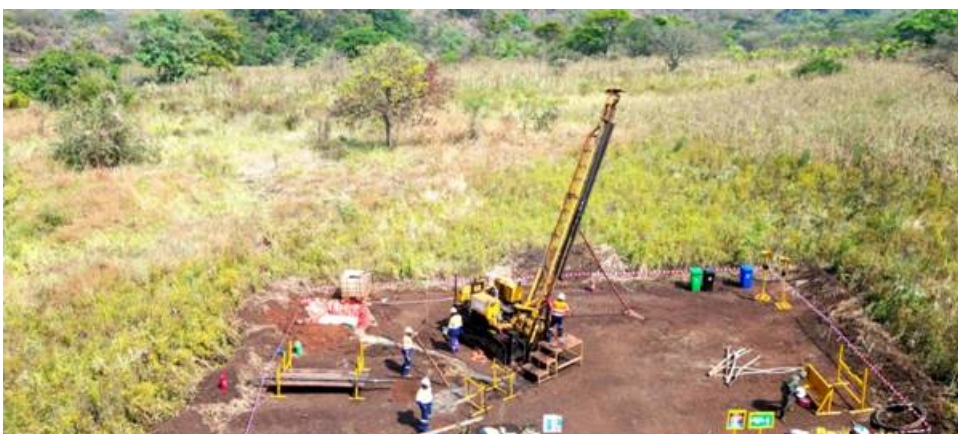
Figure 3: Rig setup and drilling the 1st Geotechnical hole
