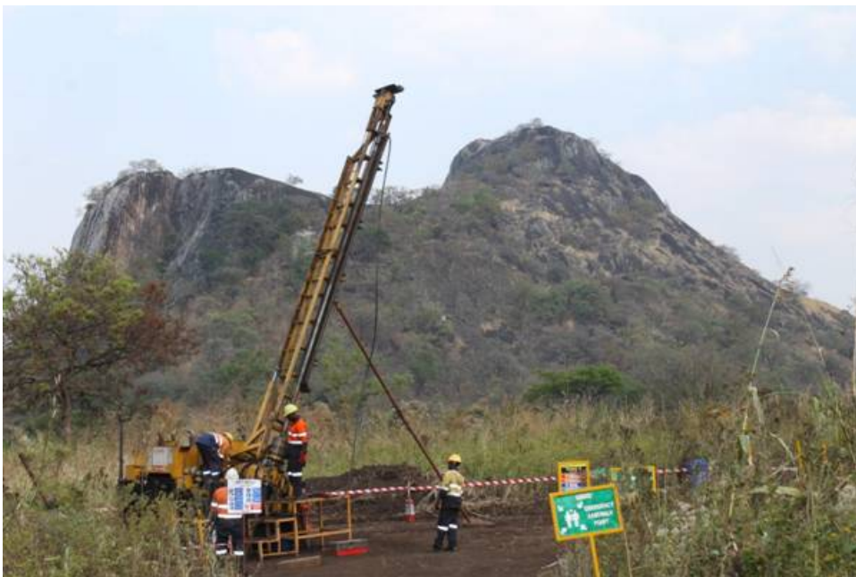
Figure 3: Rig setup and drilling the 1st Geotechnical hole
