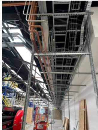
Figure 2: Gas lines being installed at Tyseley Energy Park
