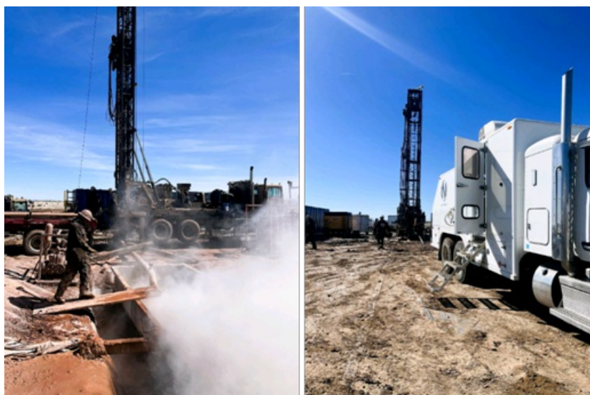
Air drilling the Lyons Sandstone Formation (left) and open-hole logging at TD (right)
