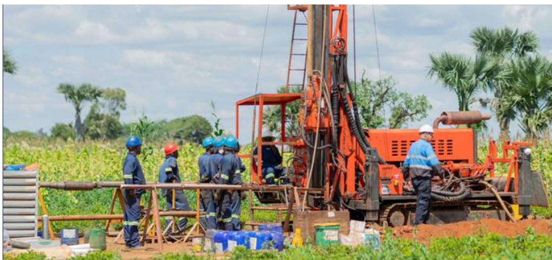
Figure 2: Geotechnical diamond drilling program underway
