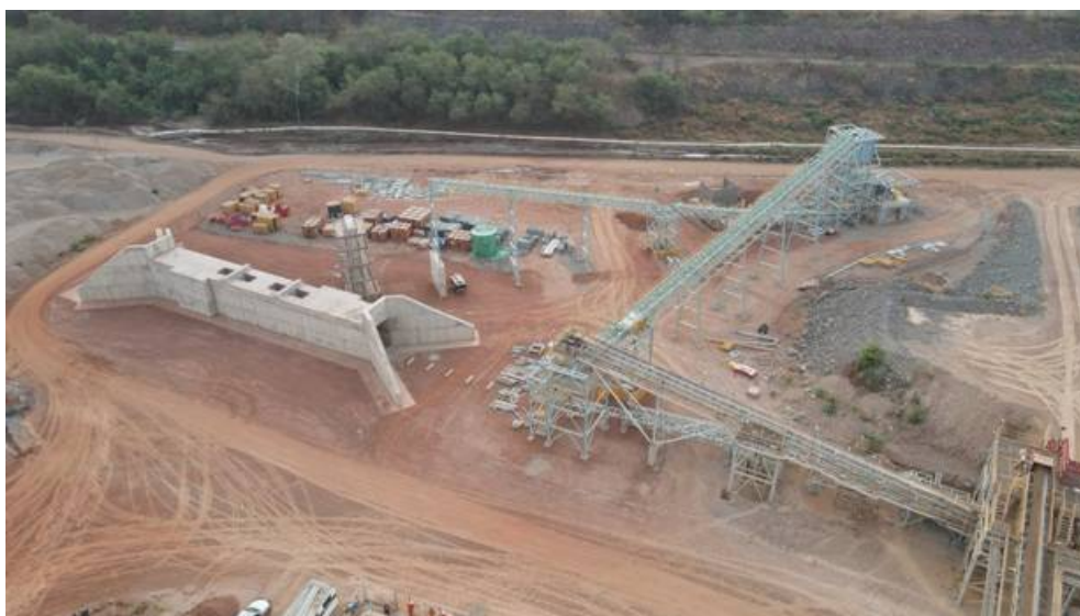
Figure 11: Secondary crusher and sulphide stockpile feed conveyor areas are 50% and 30% complete respectively
