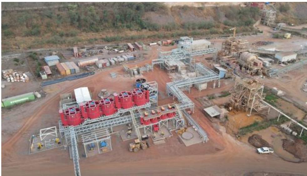
Figure 10: Ball mill and flotation areas in March under construction. The flotation circuit is now 86% complete, while the ball mill areas is 35% complete
