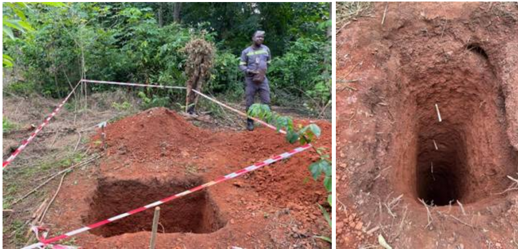
Figure 2: Example of pit hole of 1.25 metres by 80 centimetres and 5 metres depth.
