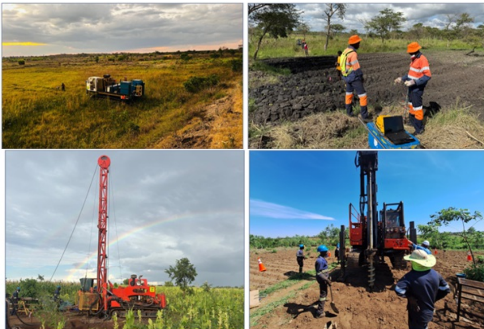
Figures 3-6 Clockwise from Top Left: Geotechnical diamond drilling, auger drilling, seismic geophysics testing using multi-channel analysis of surface waves (MASW), Cone Penetration Test with pore pressure measurements (CPTu) rig.
