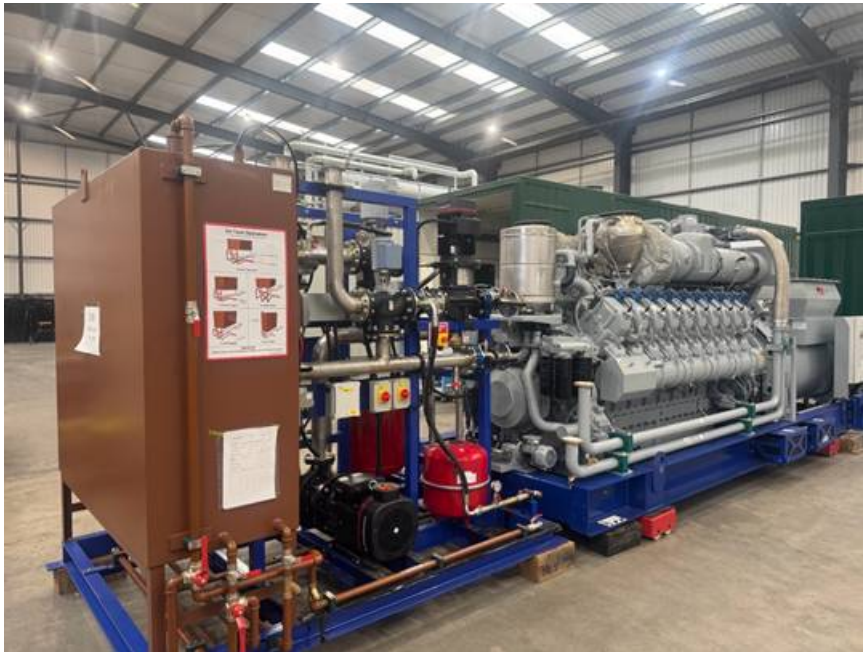
4: Fully assembled Rolls-Royce engine and cooling skid destined for Hindlip site
