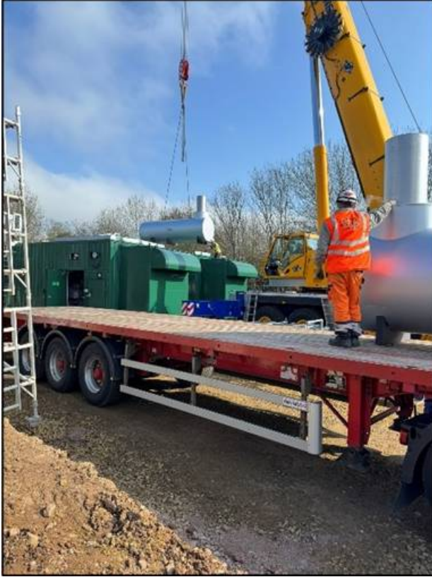
1. Rolls-Royce MTU containerised gensets delivery - being crane-lifted onto site
