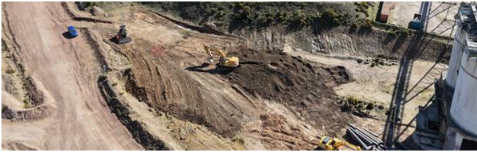
Preparatory Earthworks Underway at the Hemerdon Mine
