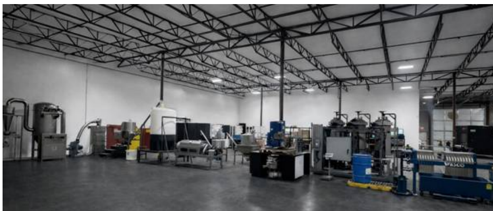
Fig. 1: Empower Lithium Processing Facility in Dallas, Texas
