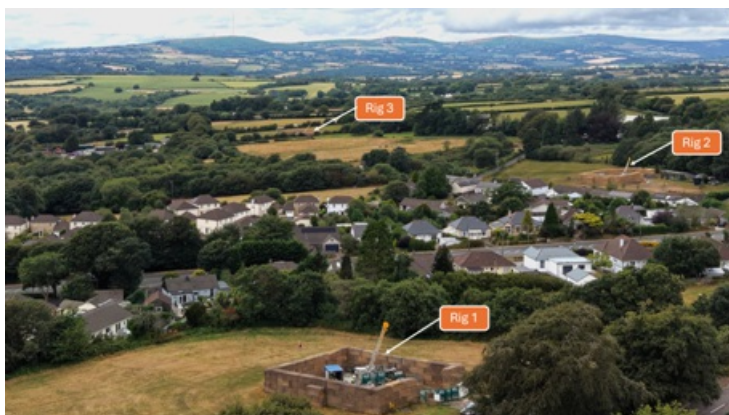
Figure 1: View looking West including Rigs 1-3 of the drilling programme, with pads fully established and drilling underway.
