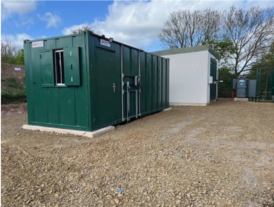
4. Completed control room and switchroom buildings
