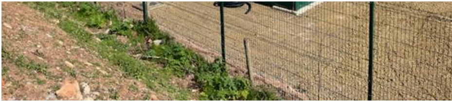
3. Completed site showing control room, acoustic fencing and gensets
