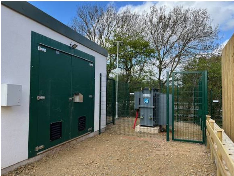
2. Completed HV switchroom and energised NGED transformer compound
