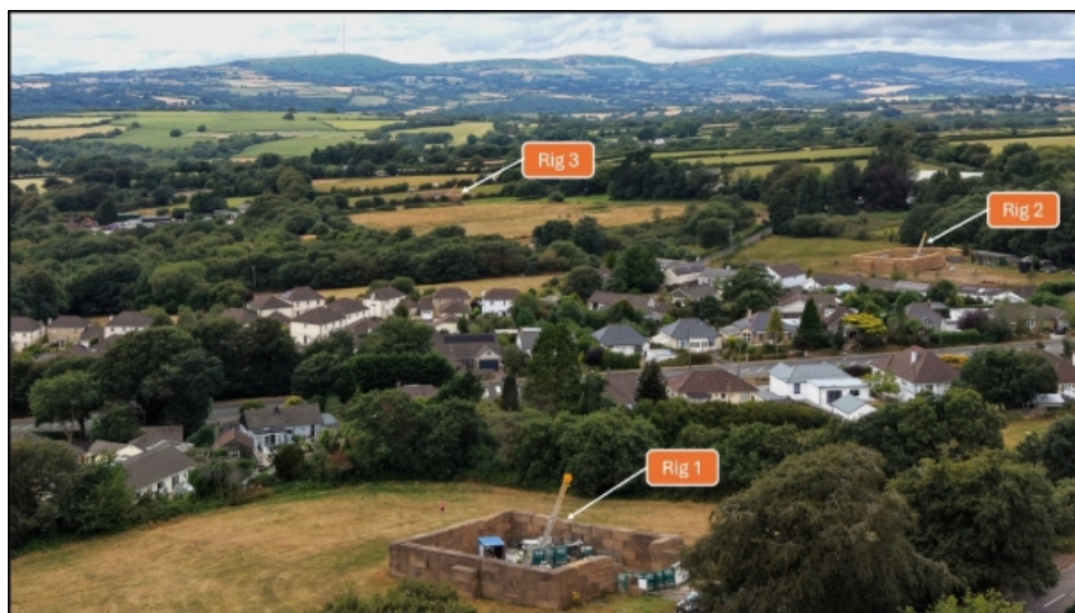
Figure 5: Locations of the three drill rigs currently operational at the Redmoor site.
