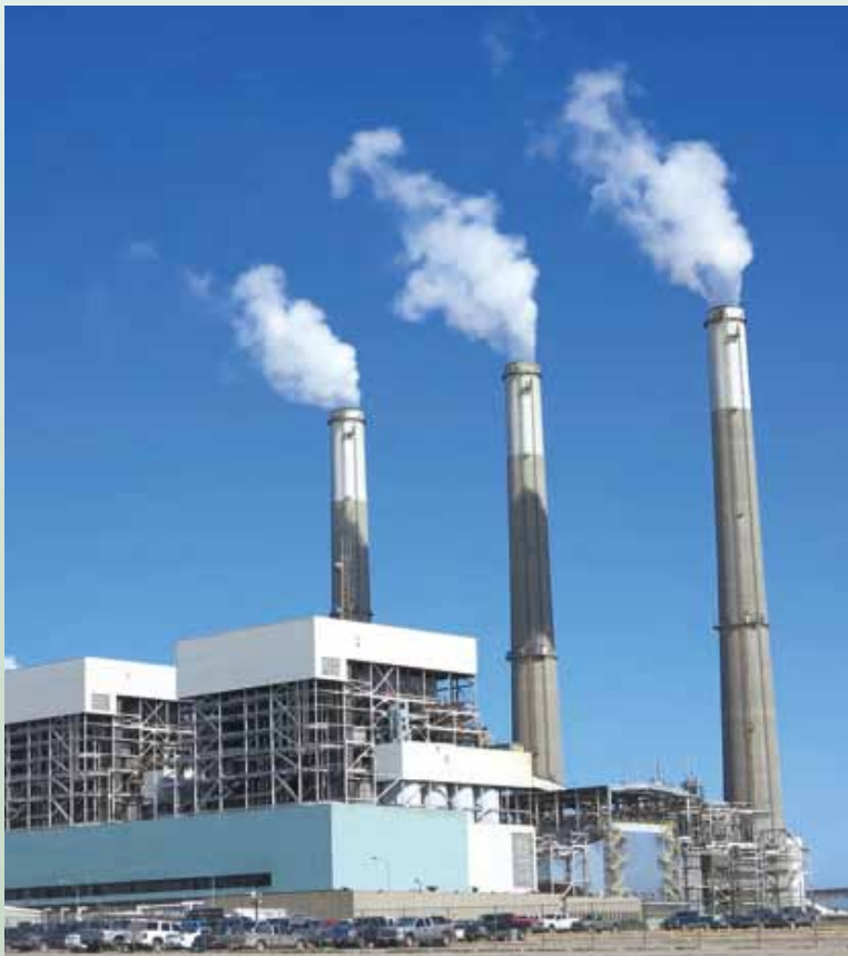
The first retrofitting project of low-NOx combustion furnaces completed in the USA 完成在美首個鍋爐低氮燃燒改造項目
