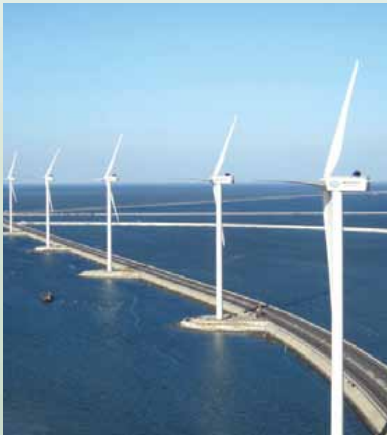
The on-grid connection of the first batch of 3MW wind turbines on land made in China 首批國產陸地型3MW風機併網
