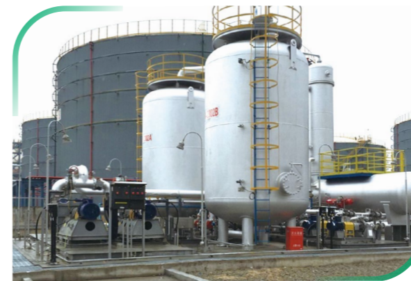
Exhaust gas treatment facilities in Ningbo Zhongjin Petrochemical's tank zone
