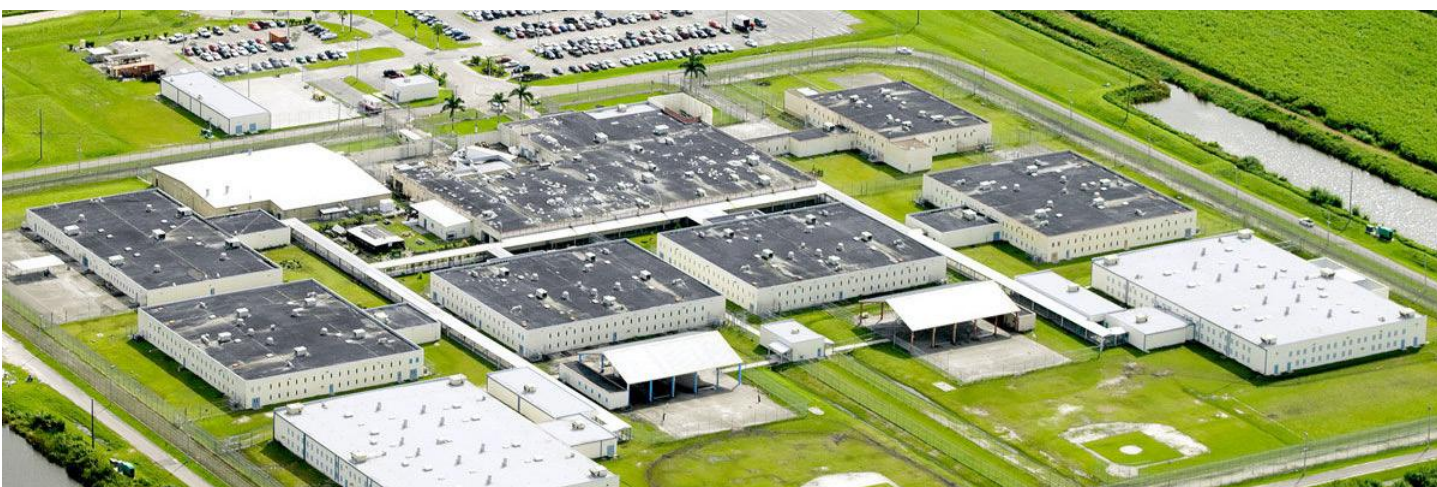
1,948-BED SOUTH BAY CORRECTIONAL AND REHABILITATION FACILITY
