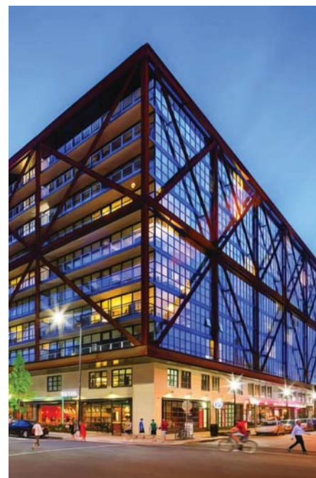
Atlantic Plumbing (multifamily asset)
