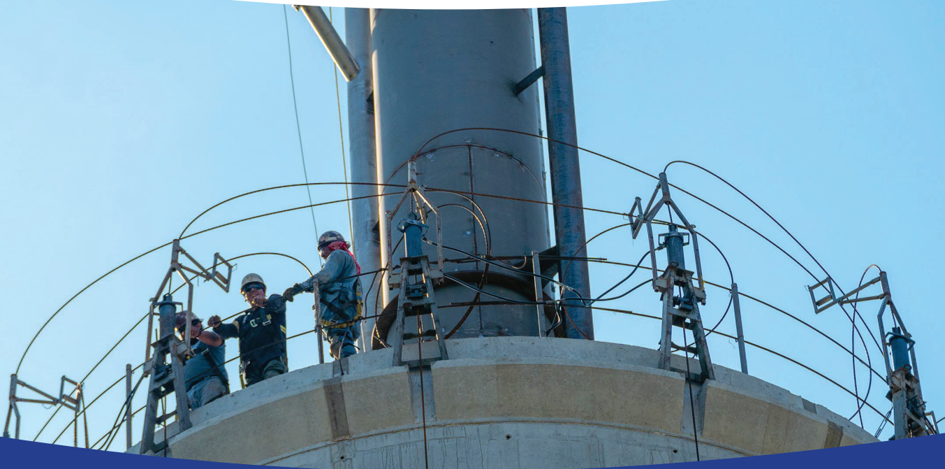
TWC's Alnwick water storage tank under construction.
