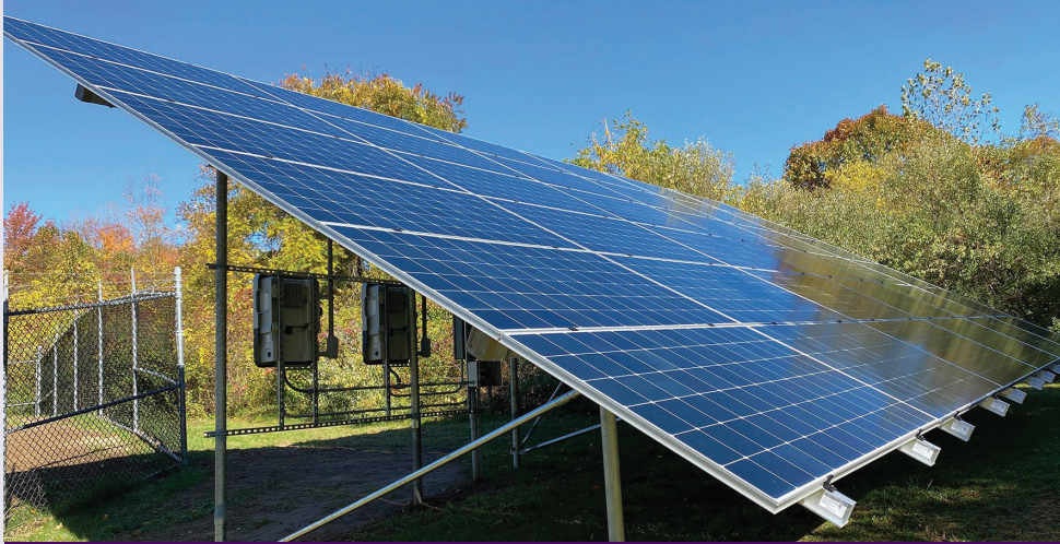
Colchester, CT — Connecticut Water completed the installation of solar panels at one of its smaller water systems that were sufficiently sized to fully meet energy requirements to pump, treat, and move water through the water system, effectively removing it from the power grid.
