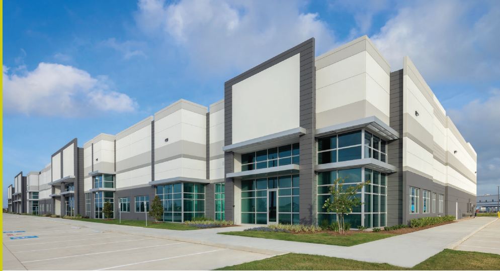
Grand West Crossing, Houston, Texas
