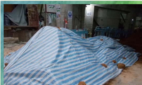
Cover the stockpile of dusty materials 覆蓋易生塵埃的物料堆
