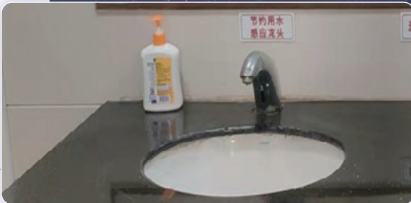
Sensor faucets are used to save water 使用感應龍頭節約用水
