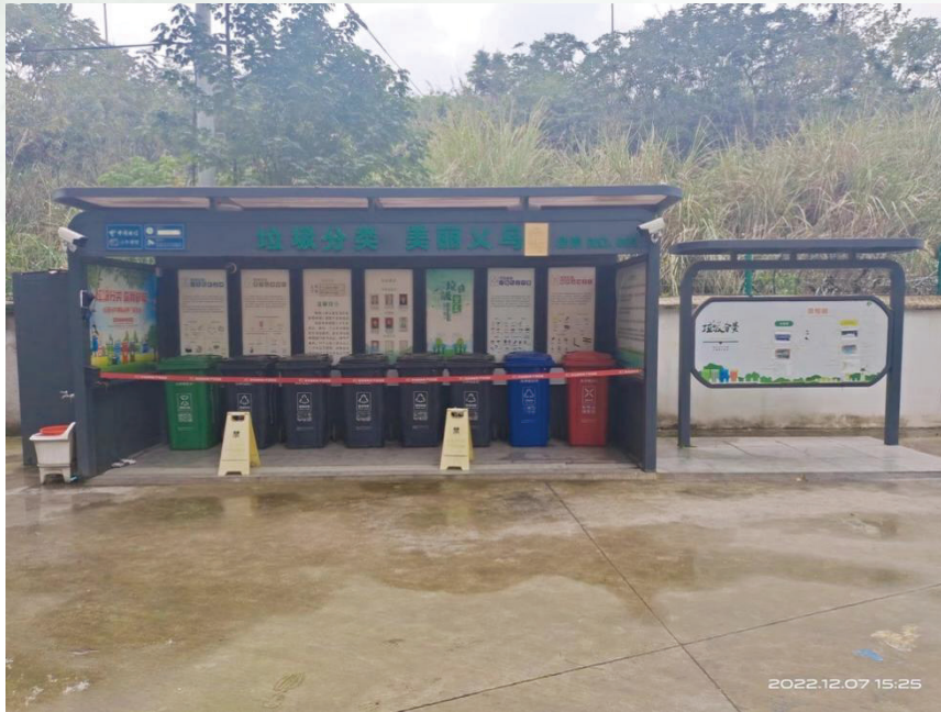
Garbage sorting station in our factories 工廠內的垃圾分類站
