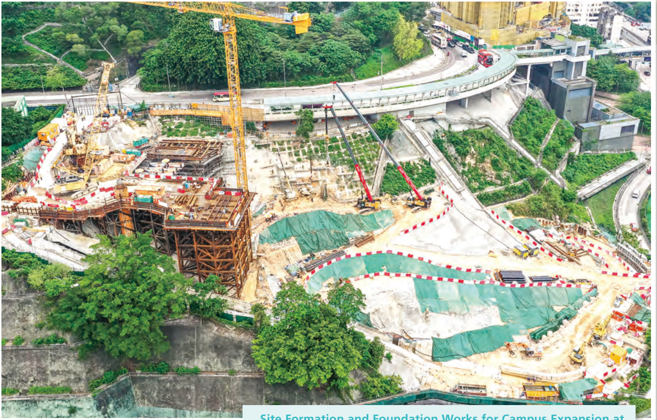
Site Formation and Foundation Works for Campus Expansion at Ho Man Tin Slope for the Hong Kong Polytechnic University 香港理工大學何文田斜坡校園擴建的地盤平整及地基工程
