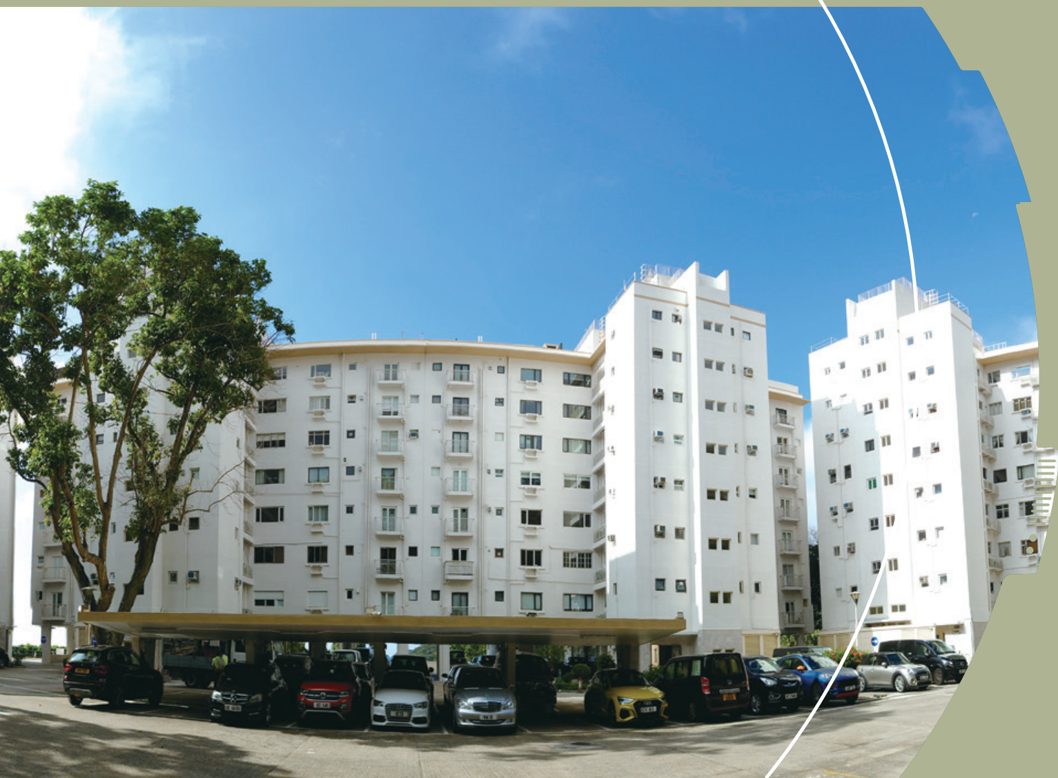
Renovation works at Carolina Gardens, The Peak 山頂嘉樂園之翻新工程
