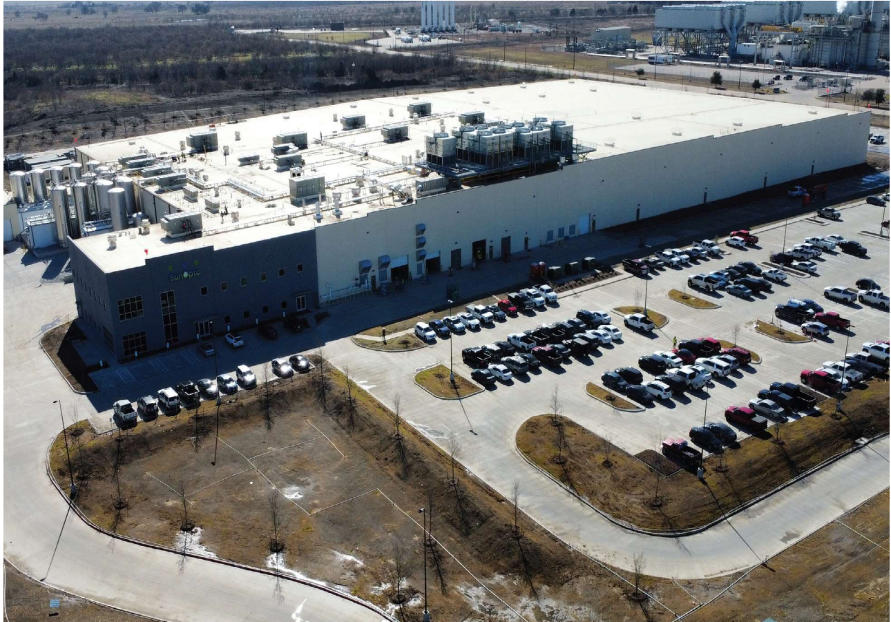
Mega facility in Midlothian, Texas
