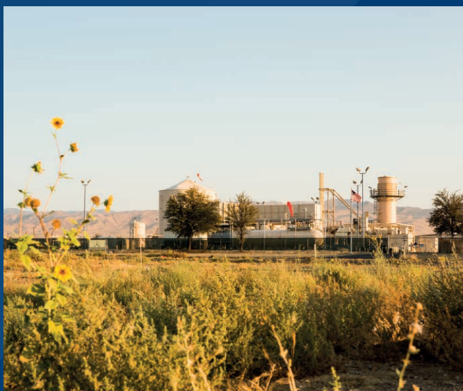
Chevron's Eastridge Cogeneration Facility // Kern County, California, United States. Photo courtesy of Chevron.
