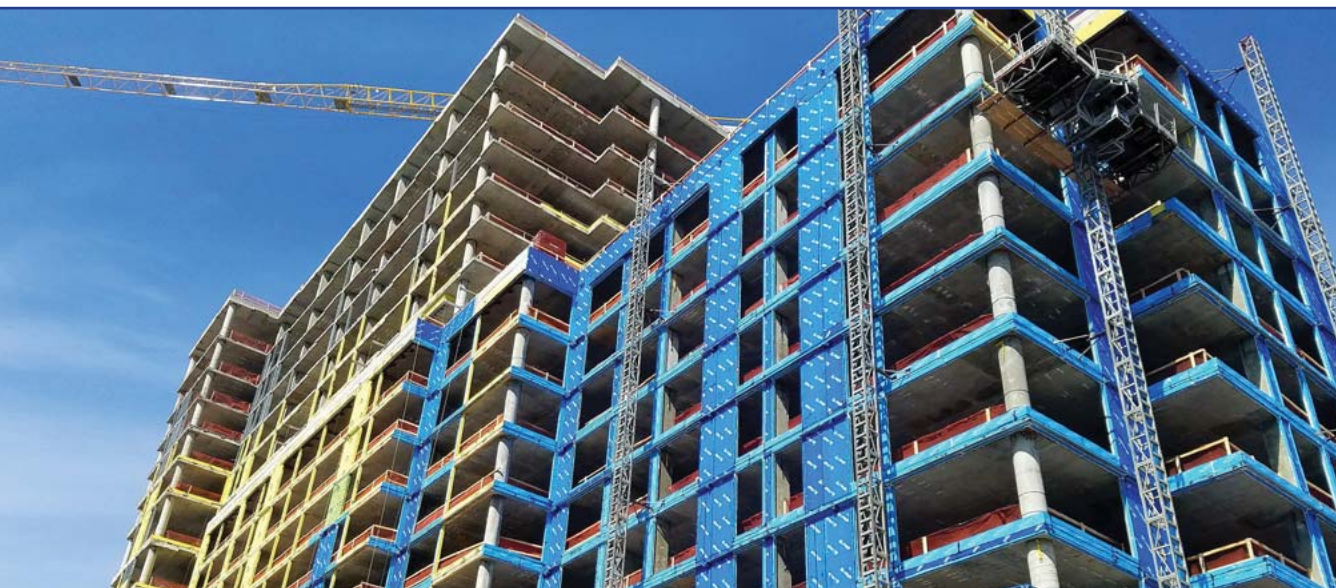
Henry Blueskin® VP160 self-adhered water resistive air barriers improve energy efficiency and comfort for building occupants
