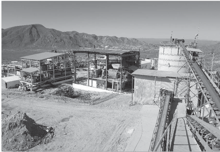
Velardeña's Oxide Plant Facility, Durango State, Mexico
