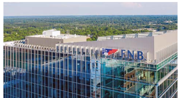
FNB Tower in Raleigh, NC, which opened in 2019, is the headquarters for our Raleigh-Durham Region.
