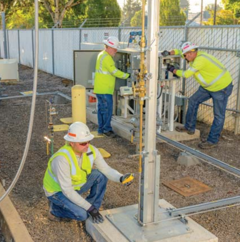
Crew performing hydrogen testing at our Sherwood facility.
