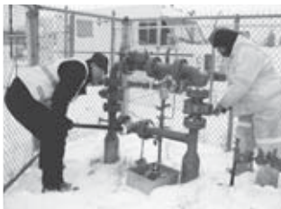
Natural gas crew, 2008.
