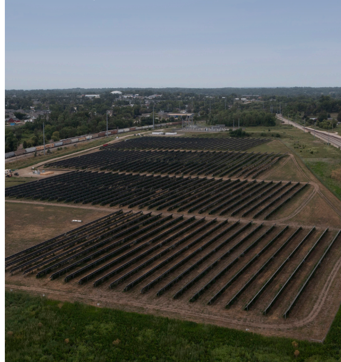
ALLIANT ENERGY COMMUNITY SOLAR – CEDAR RAPIDS, IA GARDEN
