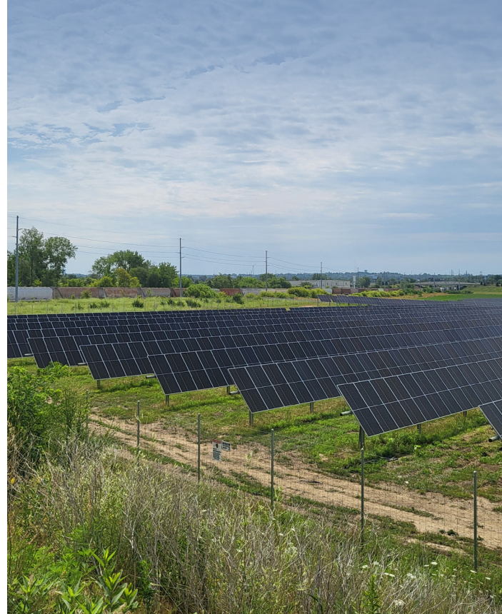
ALLIANT ENERGY COMMUNITY SOLAR – CEDAR RAPIDS, IA GARDEN
