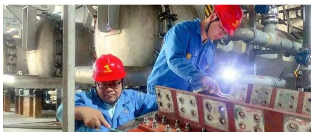
生箔车间检修生箔机电解槽阳极母板
