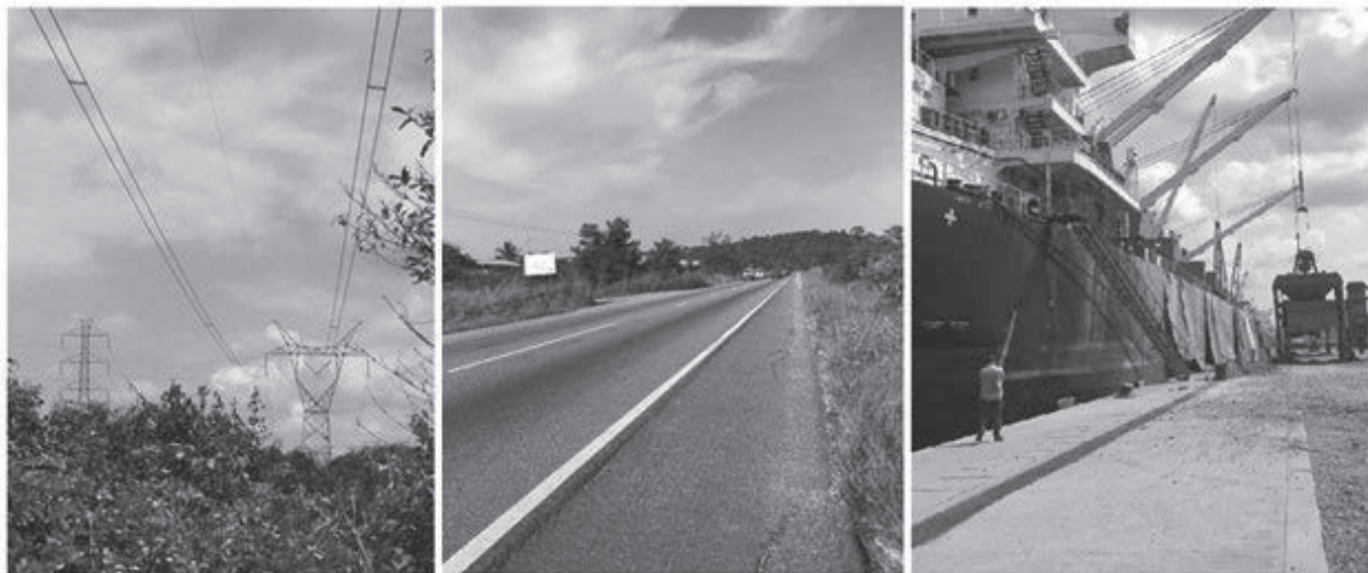
Figure 11: High voltage power transmission lines, bitumen highway and deep-sea Takoradi port close to project site.
